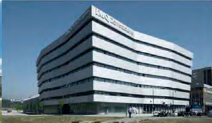
Hospital IMQ (Vizcaya)
